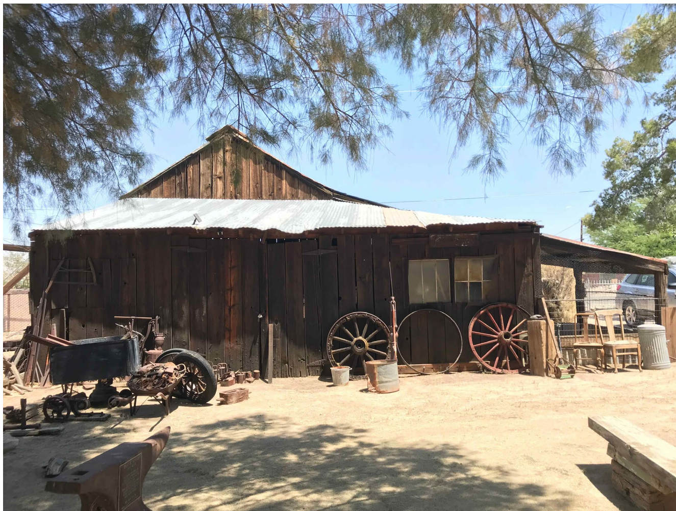
Photo 9 of 38 Alf's Blacksmith Shop, looking east at west facade.
