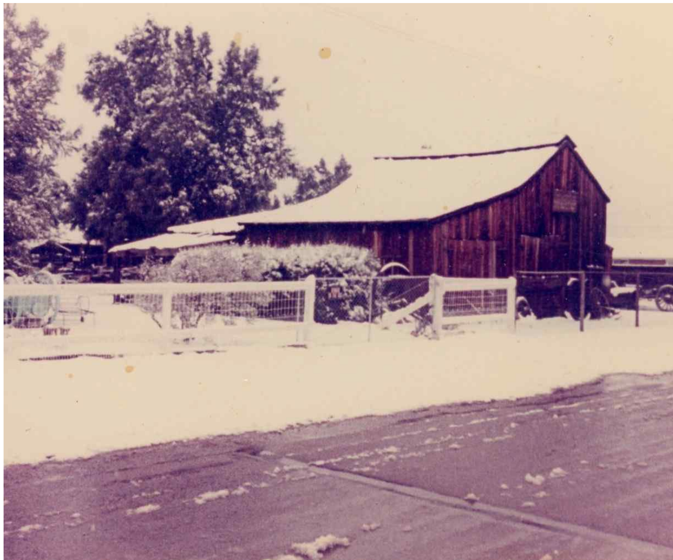
Figure 18 Alf's Blacksmith Shop in snow, ca. 1970. (Walter S. Alf Photograph Collection)
