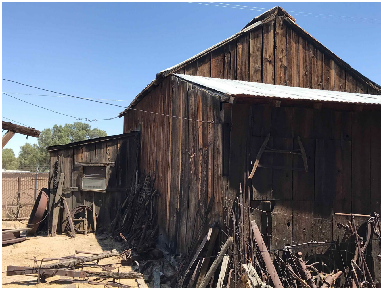
Photo 11 of 38 Alf's Blacksmith Shop, looking east along north facade.
