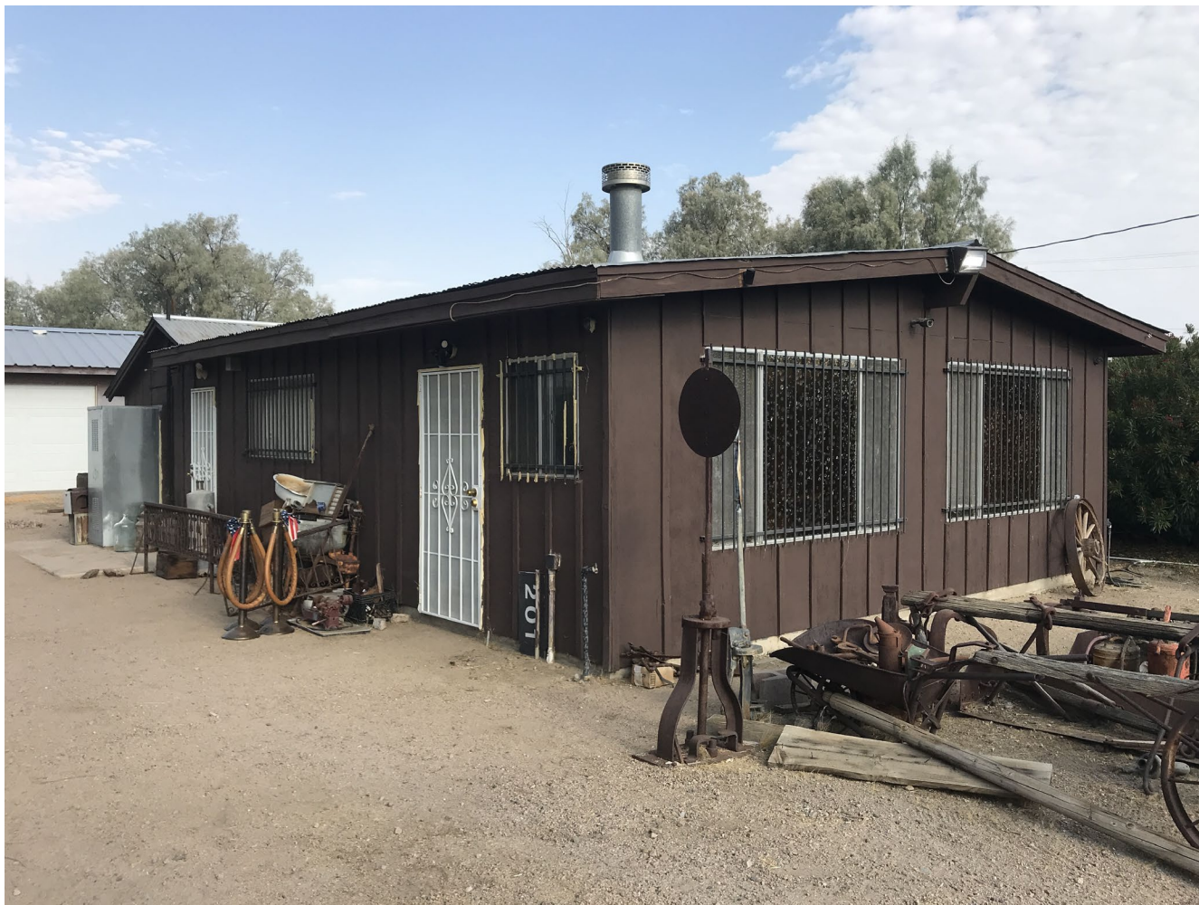
Photo 35 of 38 Non-contributing northern house, looking northwest.
