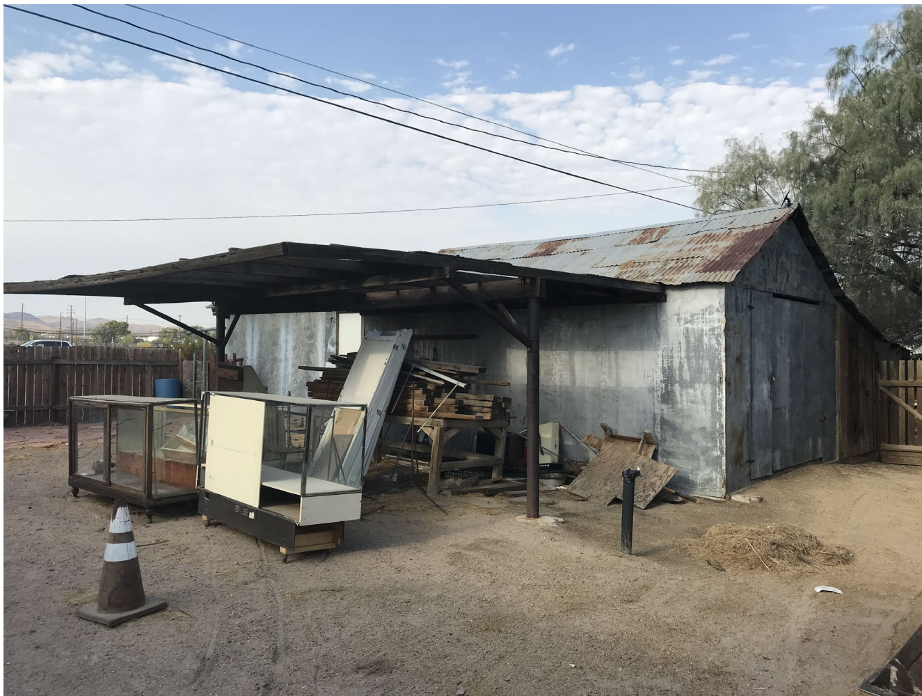
Photo 34 of 38 Non-contributing utility building, looking southwest.
