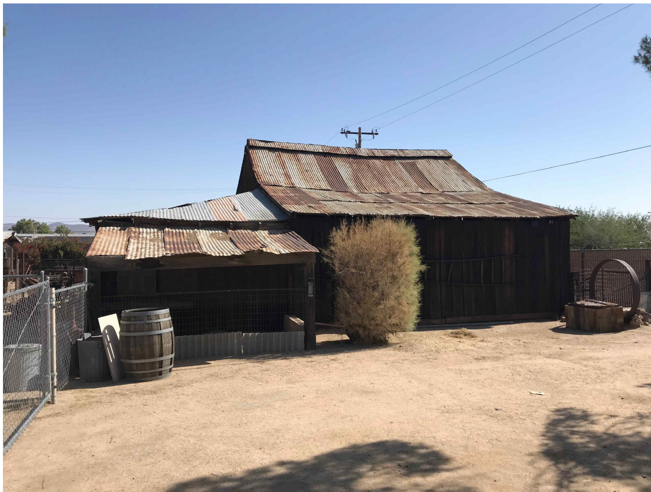
Photo 5 of 38 Alf's Blacksmith Shop, looking northeast at south facade.
