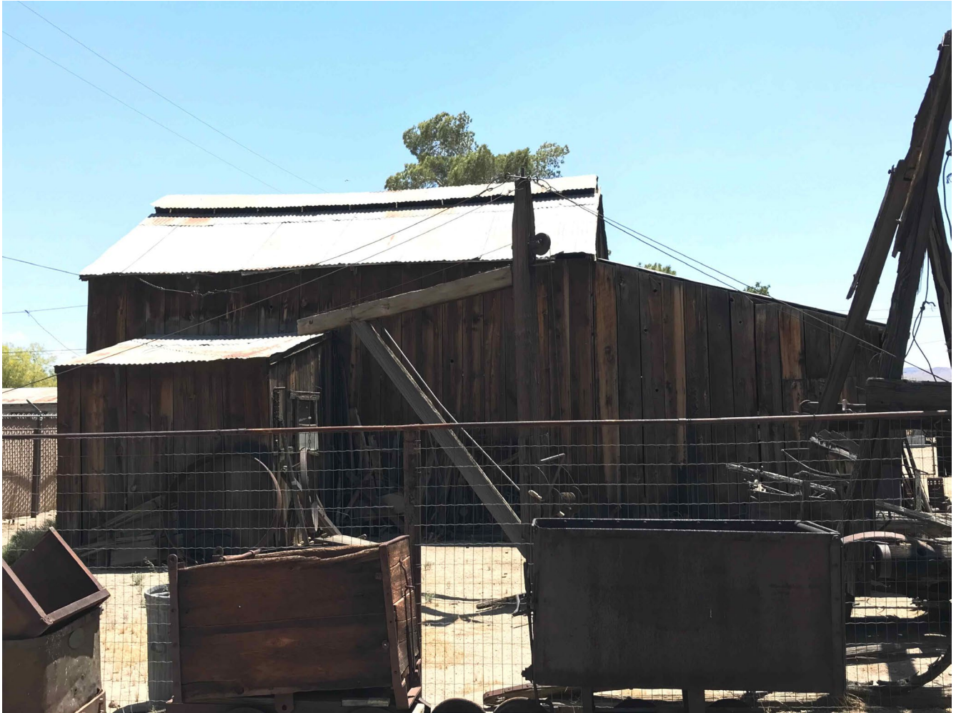
Alf's Blacksmith Shop, looking south at north facade.
