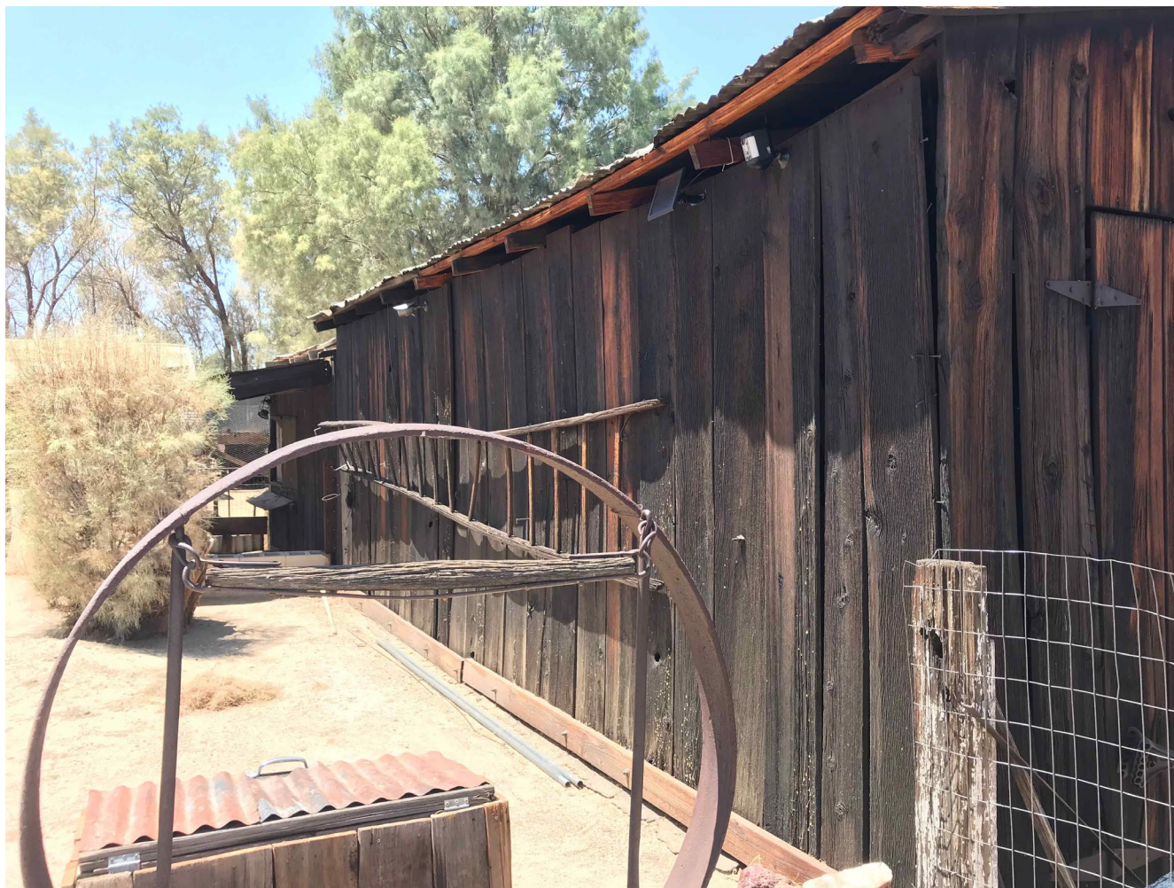
Photo 6 of 38 Alf's Blacksmith Shop, looking west along south facade.
